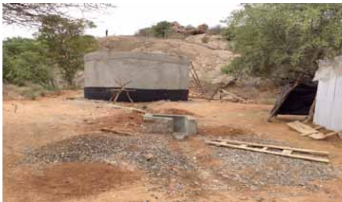
Mokori rock catchment during construction
