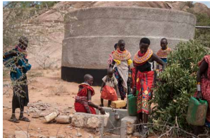
Mokori rock catchment after construction
