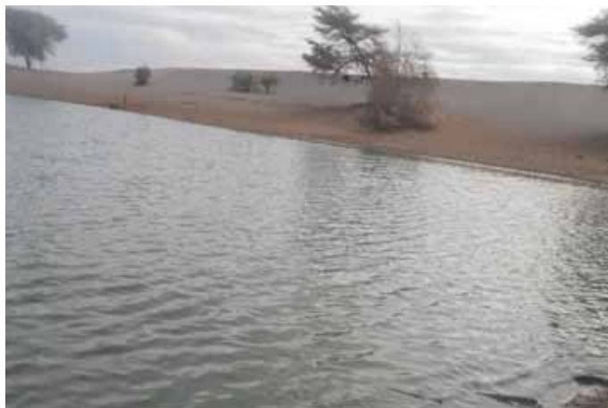
Qote Kora Water pan after rehabilitation
