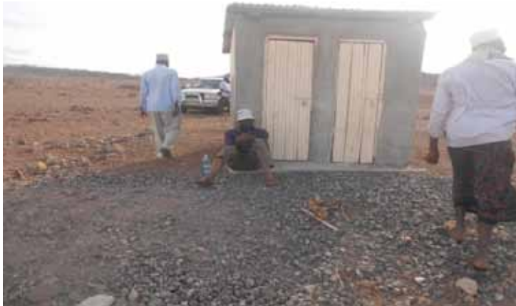
Sanitation facilities at Manyangap water pan
