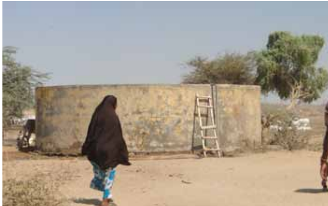
Before the rehabilitation of Yamicha Strategic Borehole
