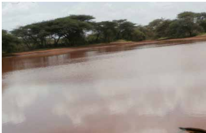
Fororsa Water pan after rehabilitation
