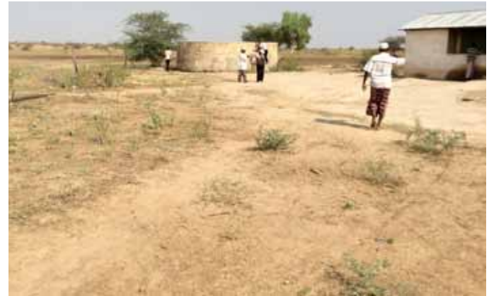
Before rehabilitation of Urura Strategic Borehole
