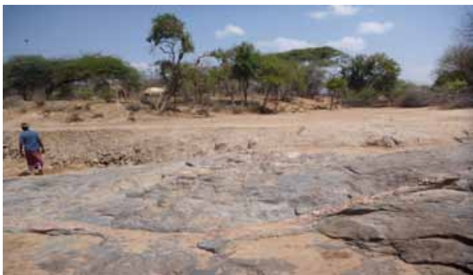
Lengiteng Sand dam before (above) and after photos (after)
