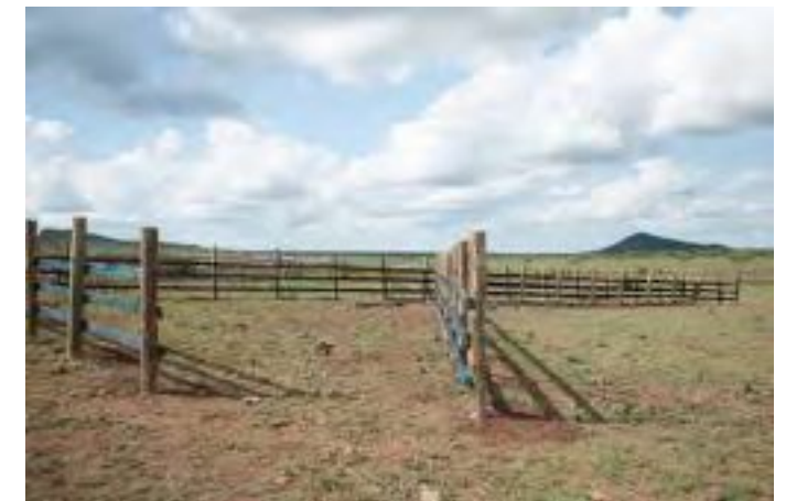
Kulamawe Livestock handling facility ICAF project
