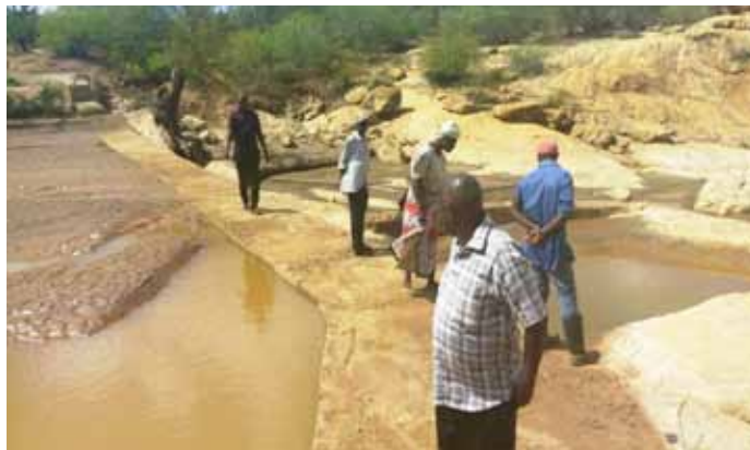
Ngai Ndethya Mega Sand dam before (above) and after (below)
