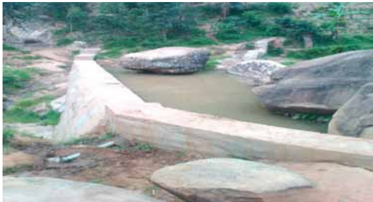
Kya aka Sand dam before (above) and after (below)
