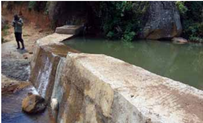
Ngutioni Sand dam before (above) and after (below)
