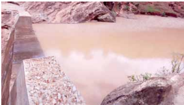
Kwa Lai Sand dam before (above) and after (below)
