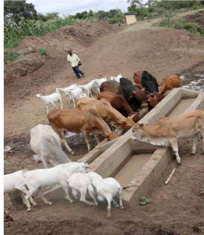
Mikuyuni earth dam
