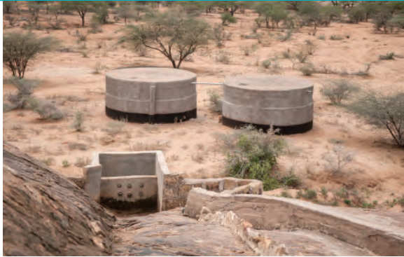
Rehabilitated Mokori rock catchment and water storage tanks in Isiolo County
