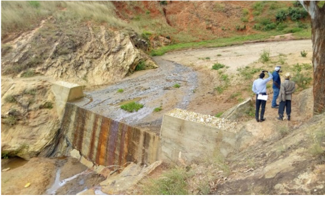
Kwa Lai sand dam, Makeni – functional © Adaptation Consortium
