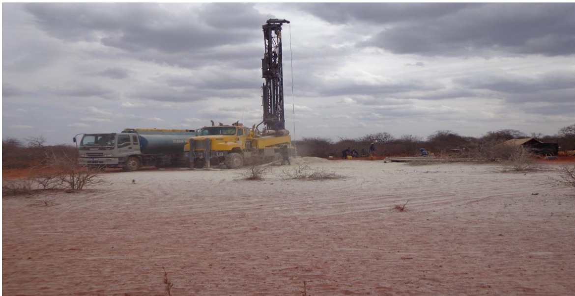
Ongoing Borehole Drilling
